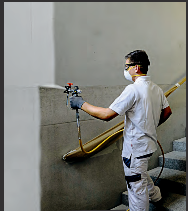
Application of fabric paint To attach fibrous material or fabrics to a wall, it is first necessary to apply a generous, even layer of fabric paint.
